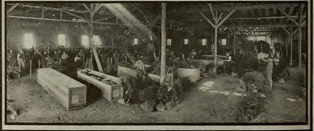
1. Sections of Propagating Houses. 2. Penna. Railroad Siding to Packing House. 3. Delivery Motor Truck. 4. Loading Shipments. 5 and 6. Sections of Packing Houses.
